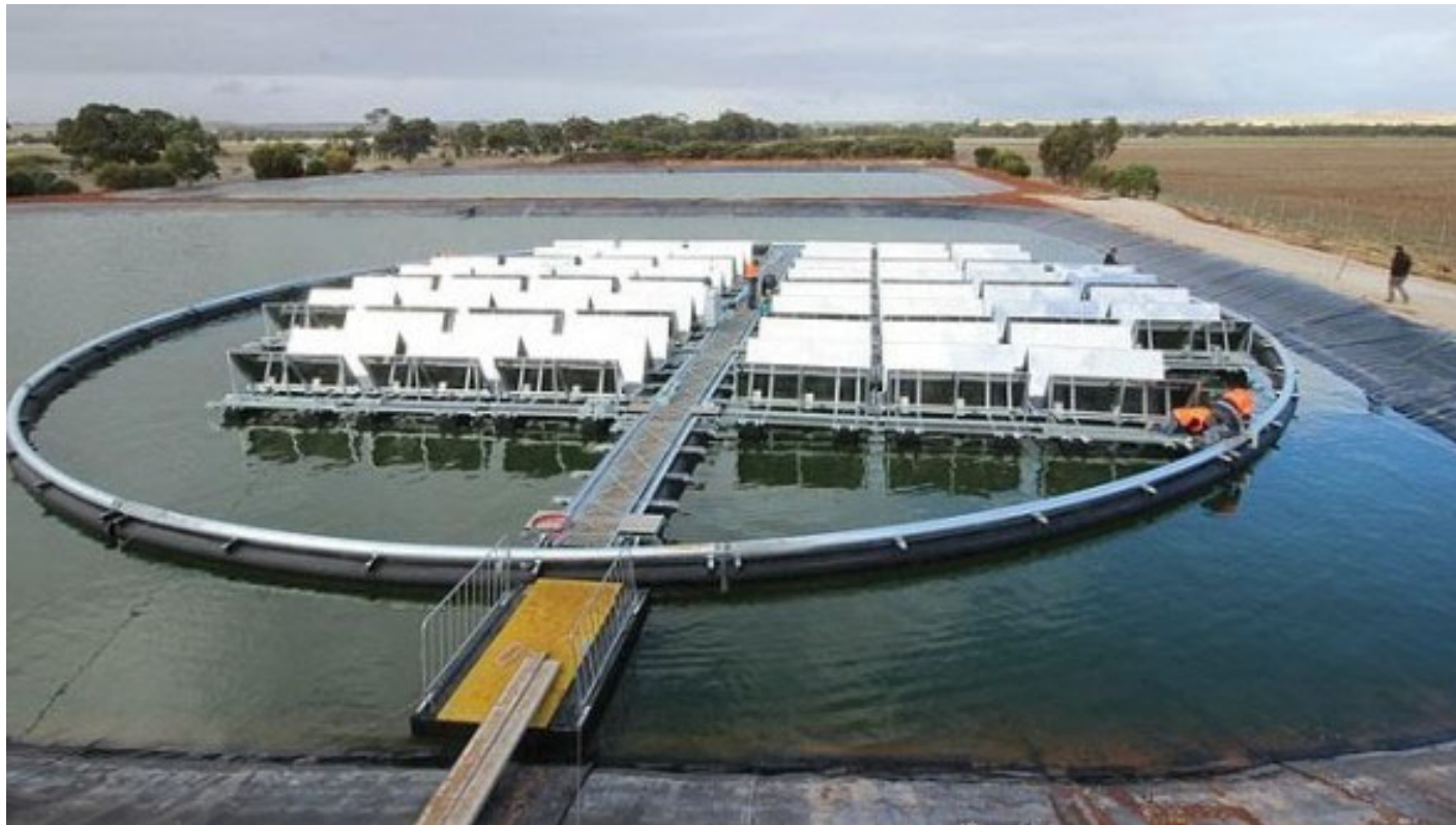
Floating solar plant at Jamestown, SA, powering the wastewater treatment facility
